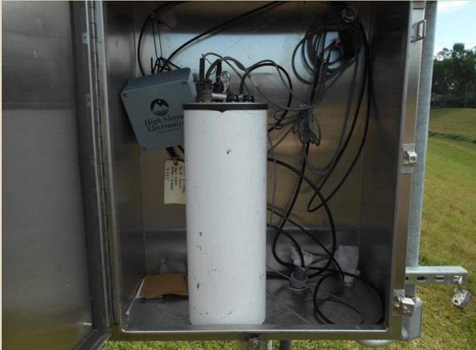
Figure 1 – The legacy ALERT configuration was cumbersome and caused unnecessary difficulty in maintenance. Included in the conversion effort was improvement to enclosure configuration.
