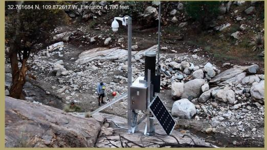
JE Fuller finished installing this new combination ALERT precipitation/stream and PTZ camera station on September 14<sup>th</sup>, 2017. This station was installed to provide advance indication of flooding from the Ash Creek Watershed which was recently burned by the Frye Fire that consumed over 48,000 acres in the Pinaleño Mountains of Arizona. Real-time data and camera imagery collected by this station can be accessed at https://water.azgfd.gov.
