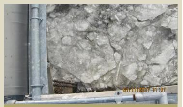
Large chunks of flushed ice are refrozen in place at Lock and Dam 18; photo credit USACE, Rock Island District
