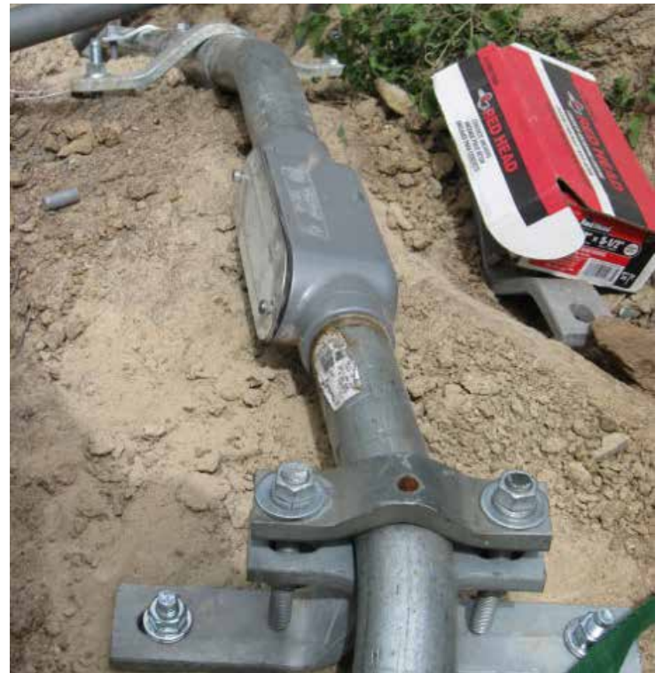
Figure 6c - Rigid conduit provides long-term protection for submersible signal cables and bubbler lines and easy access for maintenance
